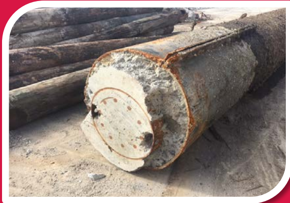
One of the steel and concrete piles after cutting
