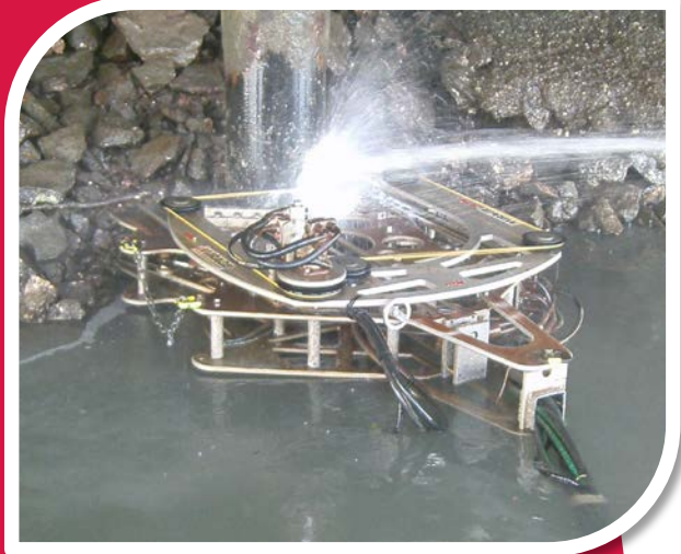
The DWS in action on the project.
